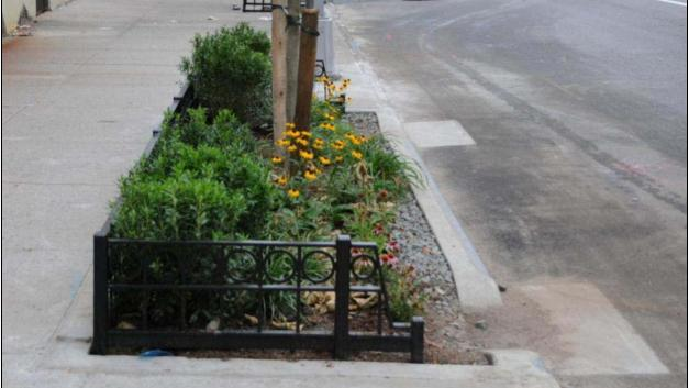
The tree pit includes the standard tree, shrubs, flowers and guard. There is also a stone buffer on the soil and a curb inlet with apron for water overflow.
