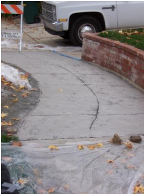
Poured in place rubber Sidewalk
